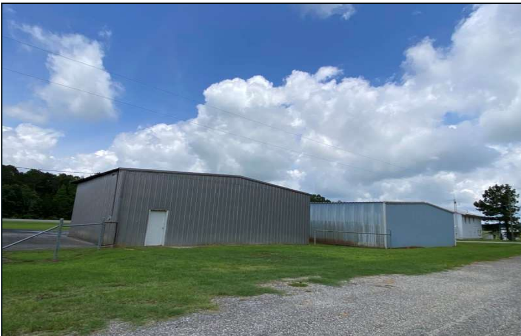
Figure 5.6. Northwest view of enclosed hangars.
