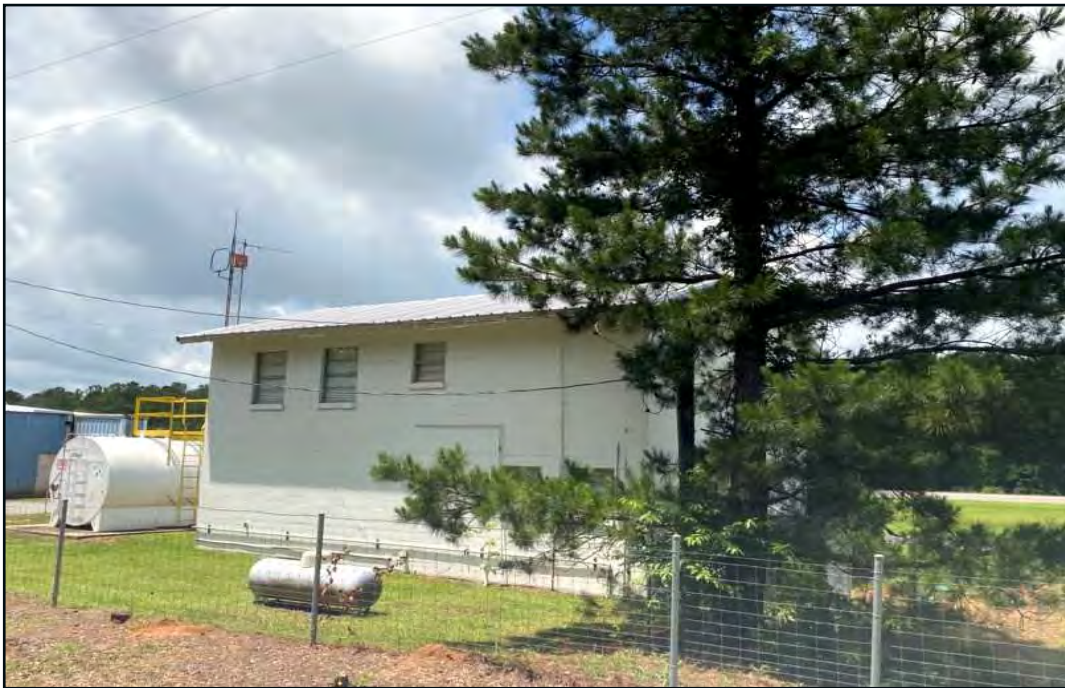
Figure 5.4. East elevation at airport office.
