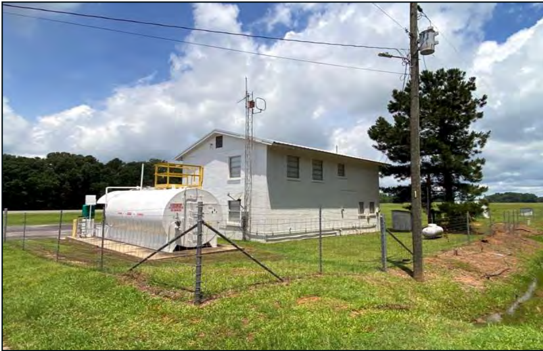
Figure 5.3. Northwest view at airport office.
