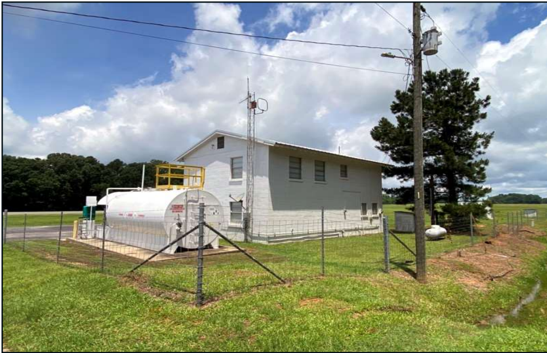
Figure 5.3. Northwest view at airport office.
