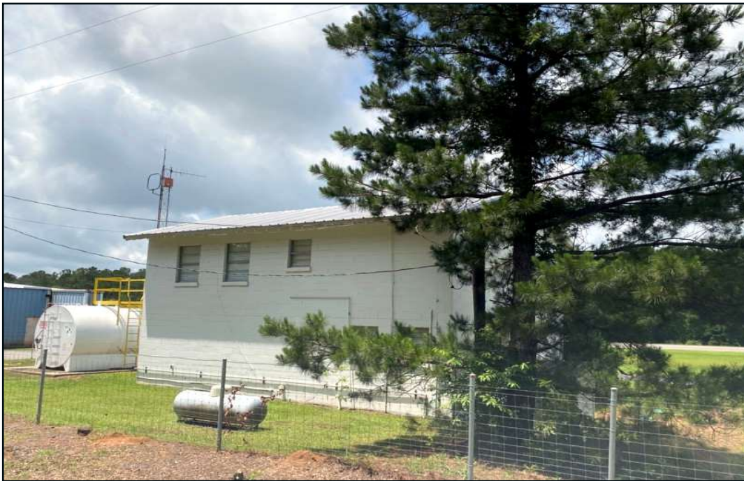
Figure 5.4. East elevation at airport office.
