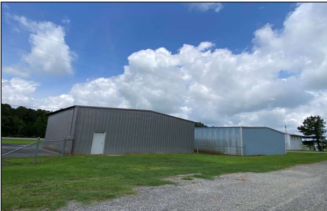
Figure 5.6. Northwest view of enclosed hangars.
